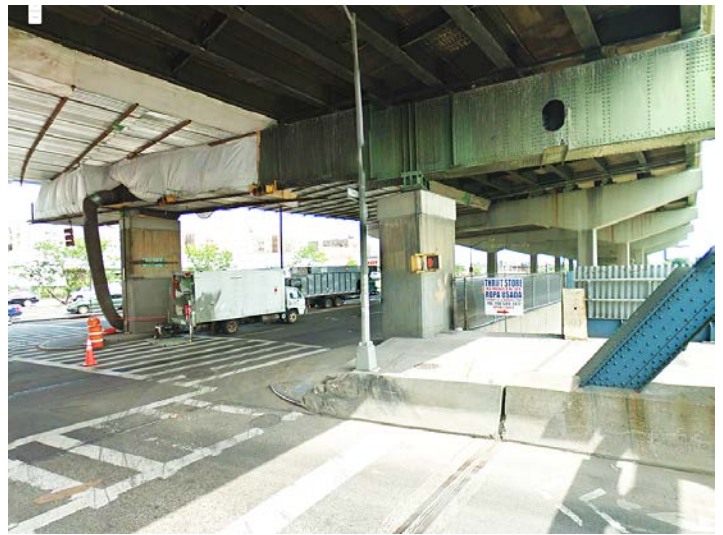
The painfully tight turn onto Bruckner. Notice the concrete barrier has been damaged by trucks that didn't turn wide enough.
